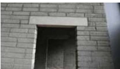
Use of Precast Lintel
