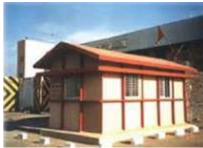
A Ferrocement Prefabricated House
