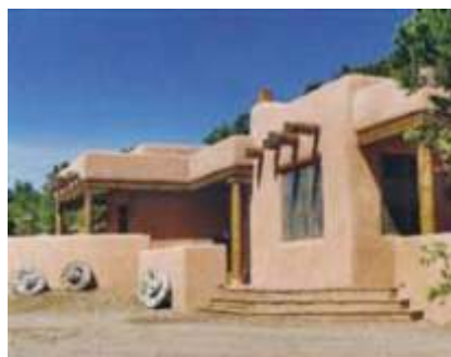
A fully finished Adobe House
